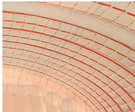
Large Scale Inflatable Structures (Market by Buildair – Conceived as a membrane-strapanchorage system to ensure the stability and functionality requirements in front of the external and internal actions)
